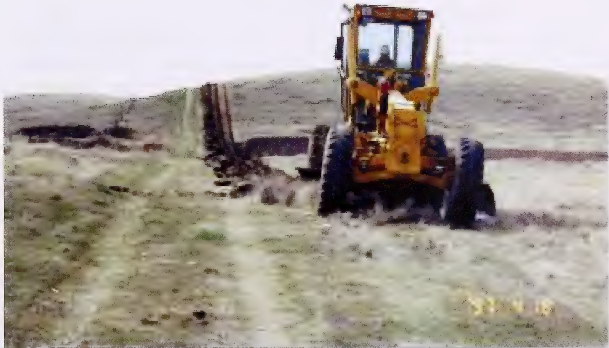
Photo 27 Blade width stripping
